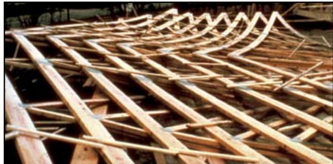
⚠️ **Warning!** Trusses are not designed to resist lateral impact loads. A falling worker attached to a single truss could cause all the trusses on the structure to collapse in a domino effect.
